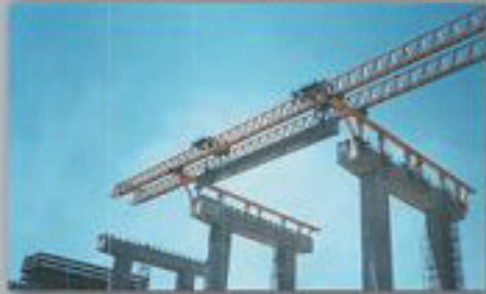
Beam Launcher 160t - Shanghai FEC
