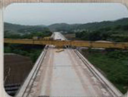
180° turning operation on deck
