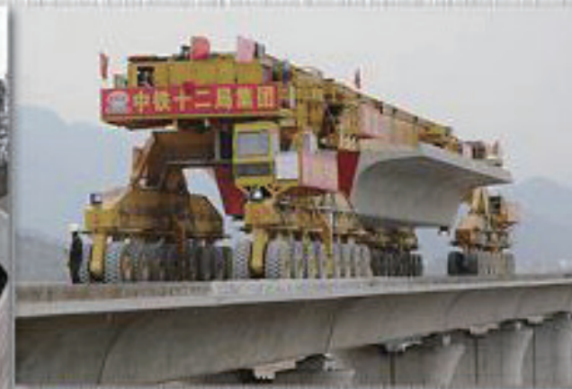
Special Launching Gantry (Passing through tunnel) in 900 ton capacity for Wuhan-Guangzhou High Speed Railway/12th BG CRCC
