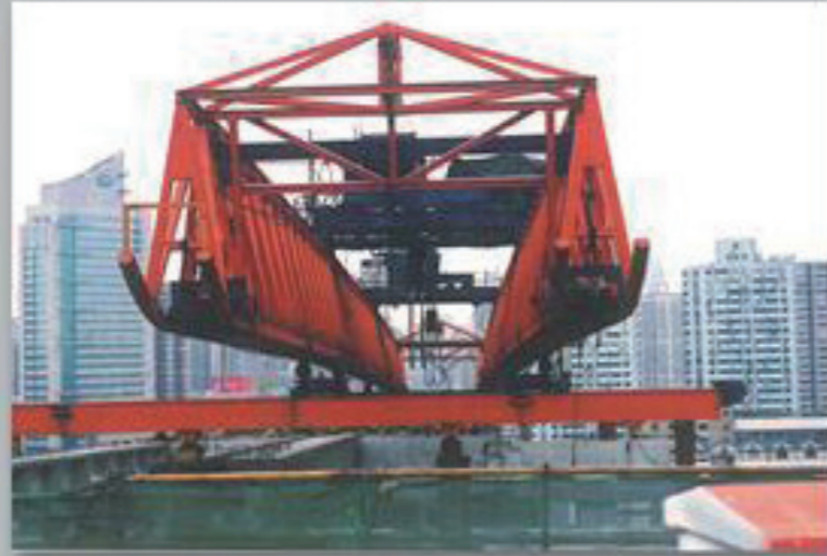
Beam Launcher 160t - Shanghai SMECO
