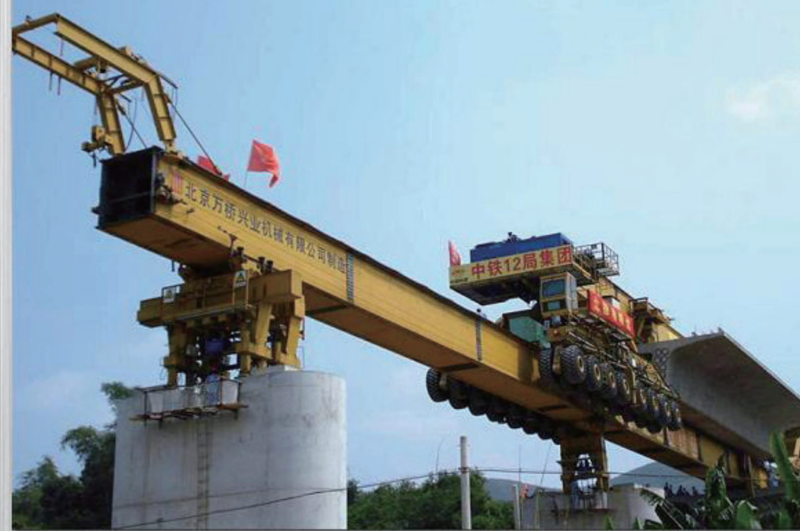
Special Launching Gantry (Passing through tunnel) in 900 ton capacity for Wuhan-Guangzhou High Speed Railway/12th BG CRCC
