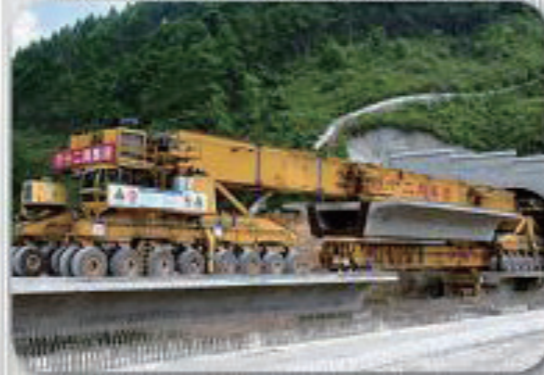
Erecting bridge at tunnel exit and entry
